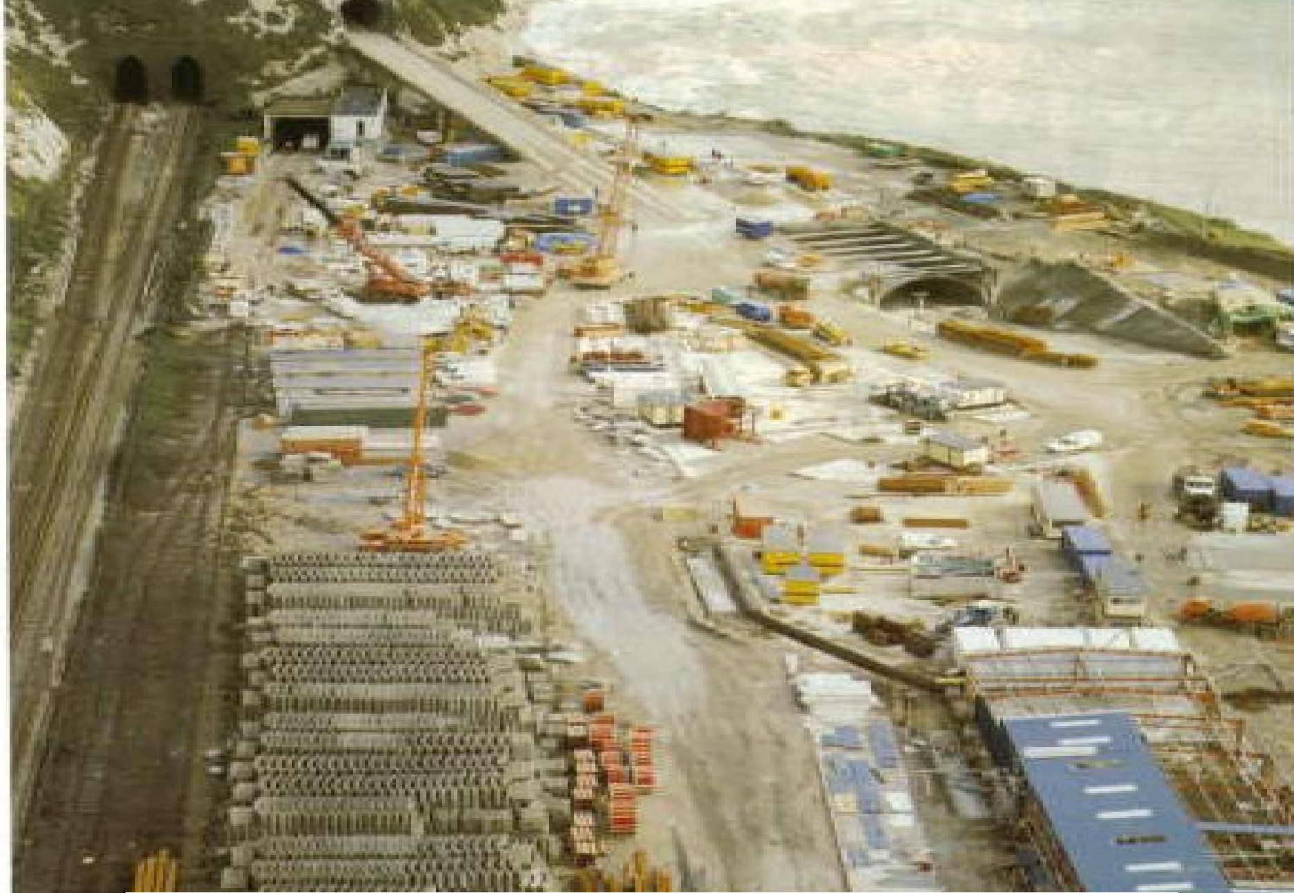
TUNNEL CONSTRUCTION ENTRANCE – UK SIDE
