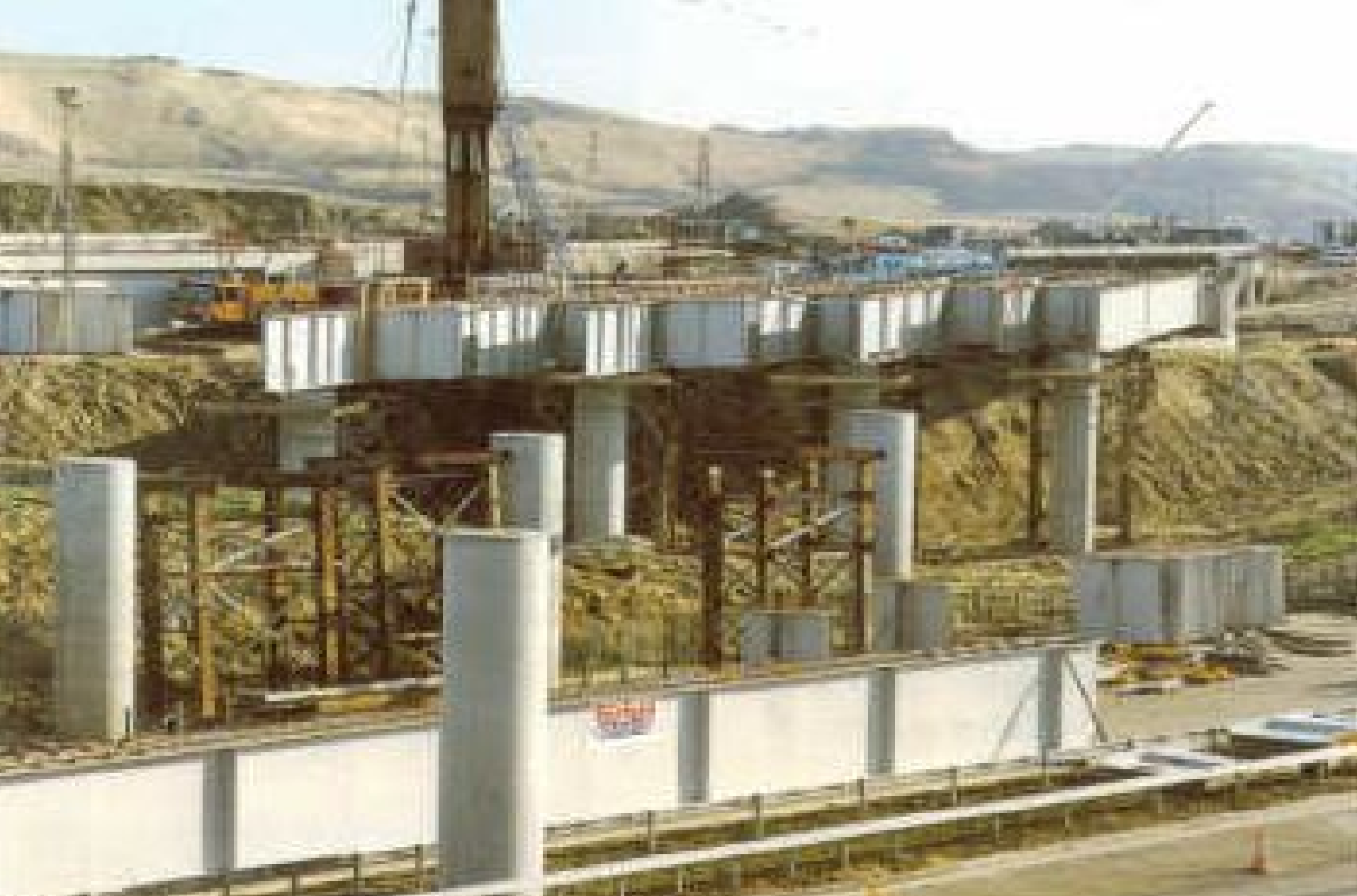
M20 BRIDGE CONSTRUCTION
