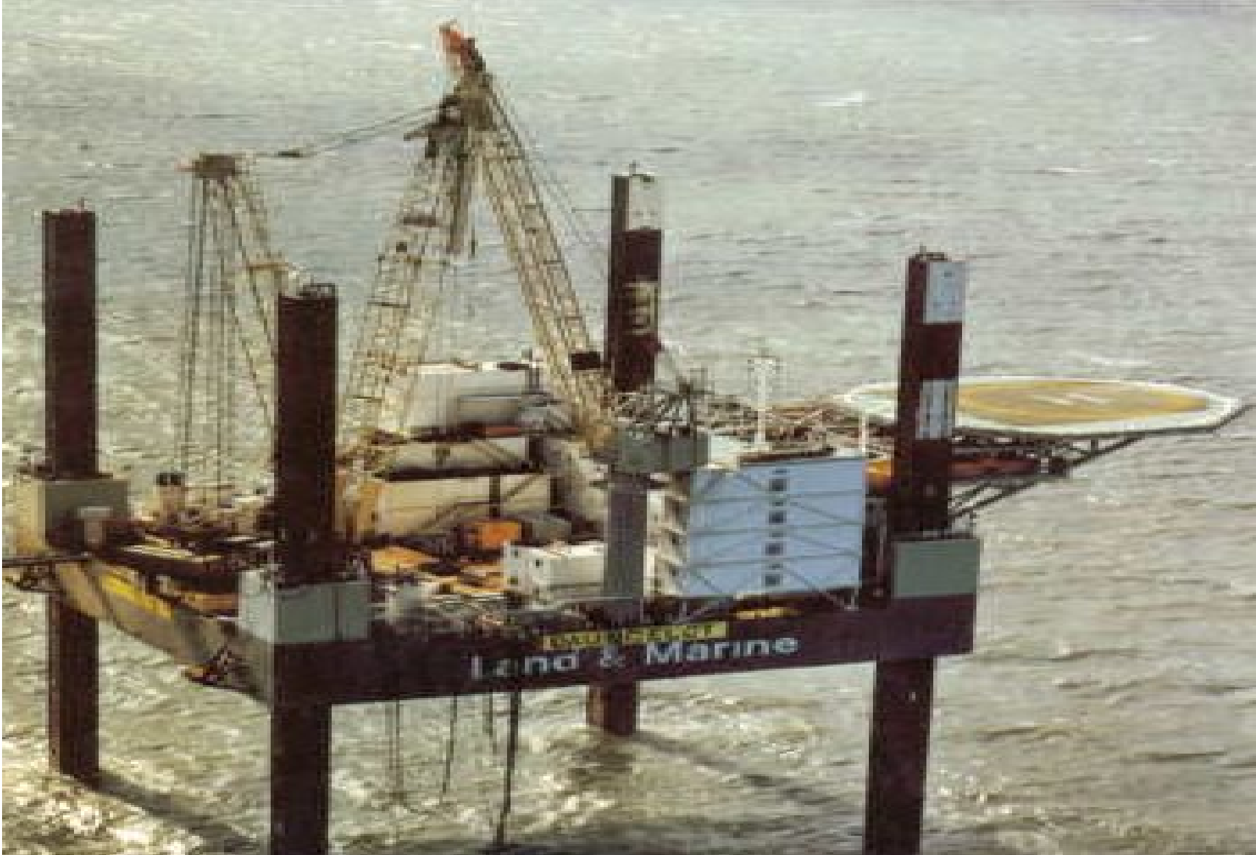
SEAWALL JACKUP BARGE
