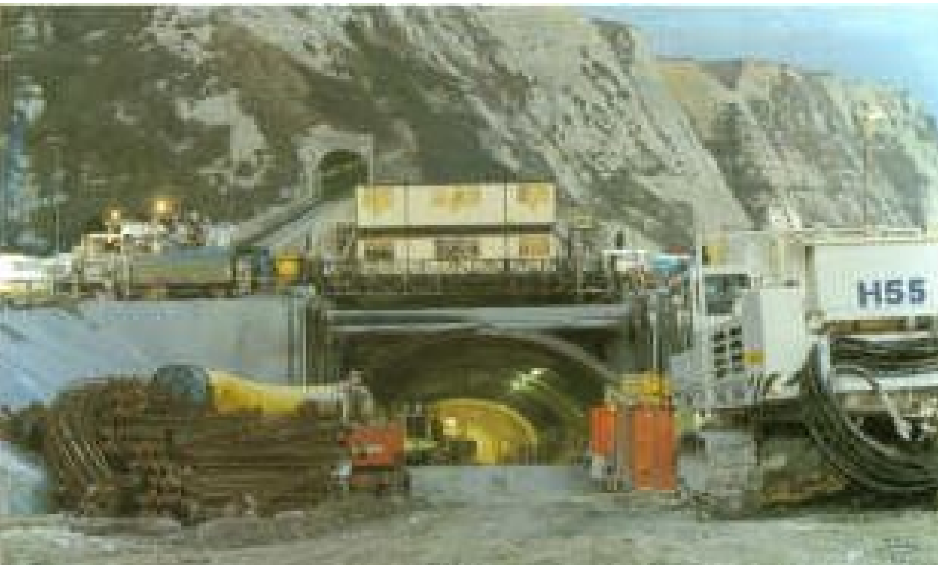
ENTRANCE ADIT – UK SIDE
