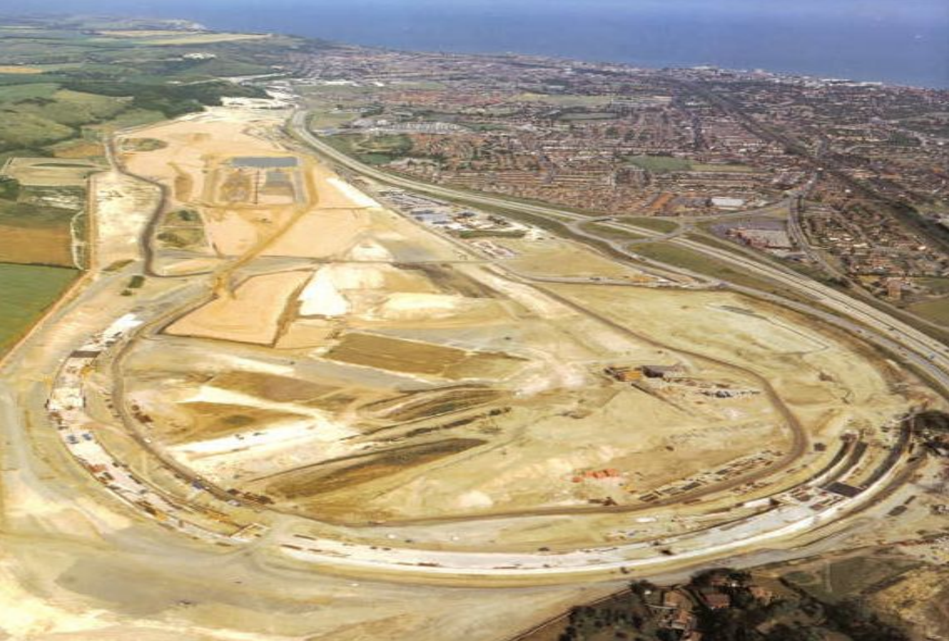
TERMINAL SITE LEVELLED – BEFORE CONSTRUCTION
